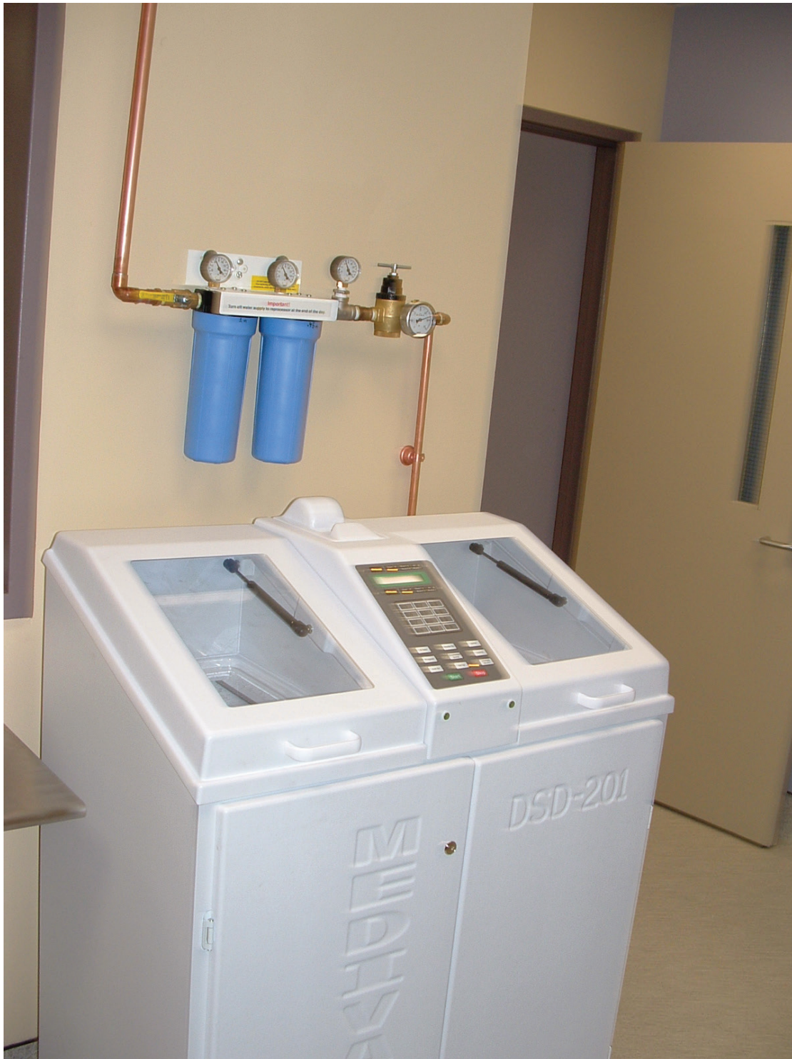
Figure 8. Sample Installation of a DSD-201LT/SSD-102LT
