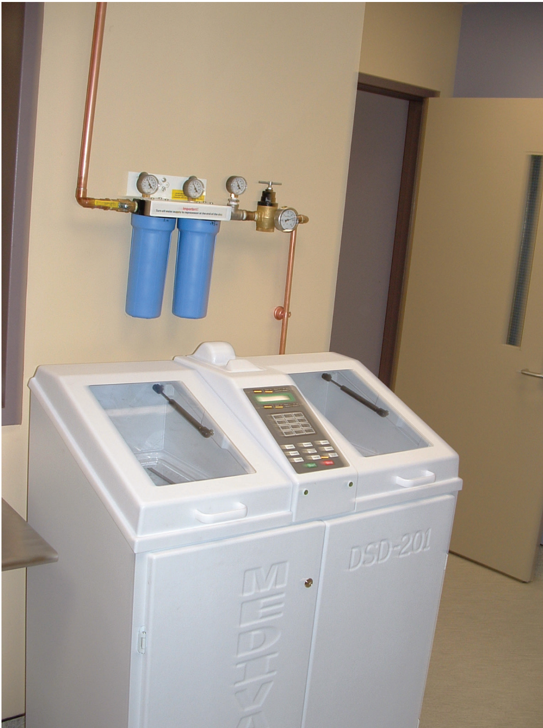
Figure 8. Sample Installation of a DSD-201/SSD-102
